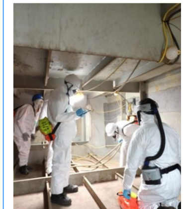
Workers in full PPE and RPE
