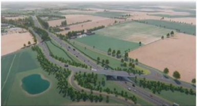
How the revamped A47 between Blofield and North Burlingham would look, according to National Highways (Image: Highways England)
